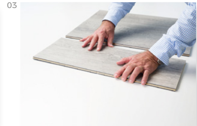
Place the planks gently on the floor
