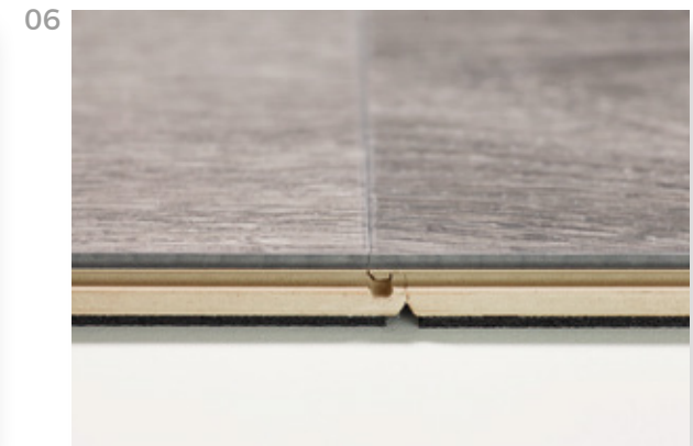
Planks are now fully inter-locked
