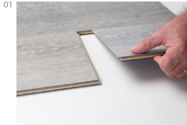
Start by engaging the plank on the long side (angle-system)
