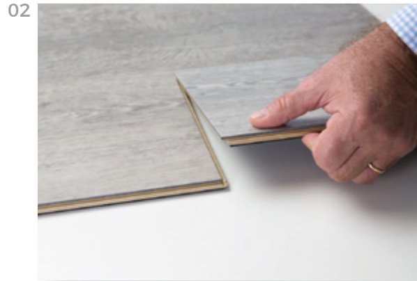
Slide the plank until it reaches the short side of the next plank
